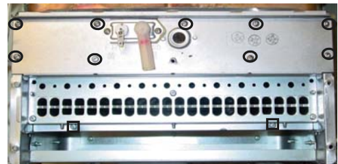
Figure 2 9 screws ○ (burner cover plate) 2 screws □ (burner)
